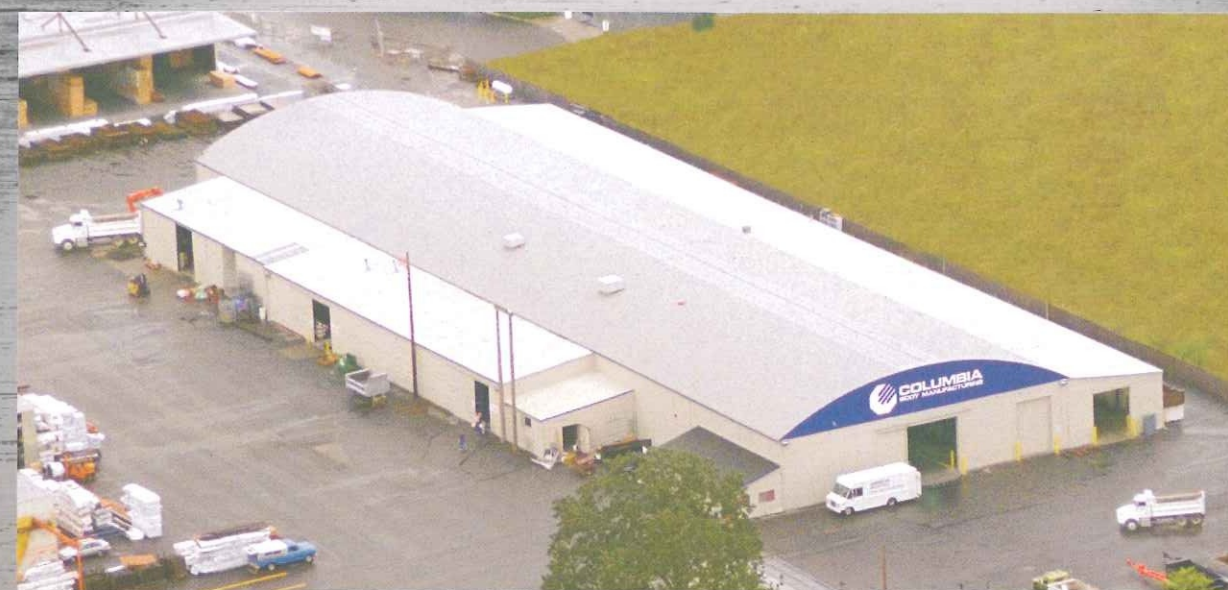
60,000 Sq. Ft. Manufacturing Facility
